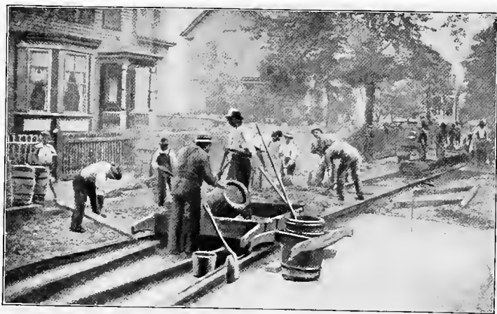
Mixing and placing concrete base.
